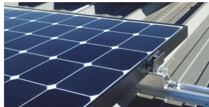
Figure 5 Installed glass faced solar PV panels showing end clamp installation.
