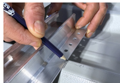
Figure 2 Mark application (bond line) area on the metal roof.
