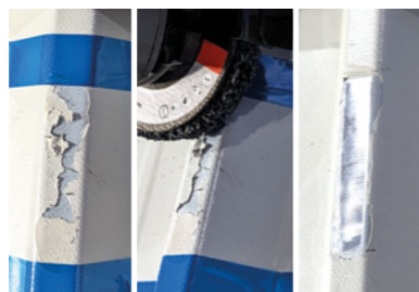
Figure 3 Grind/clean area for bonding.
