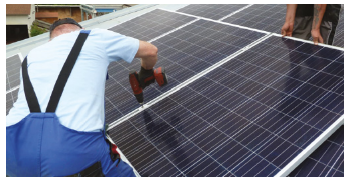
Figure 4 Installing the Mid clamp.
