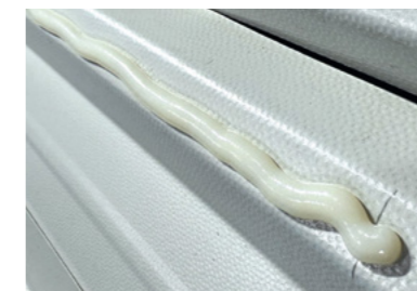
Figure 6 Apply adhesive to bond area.
